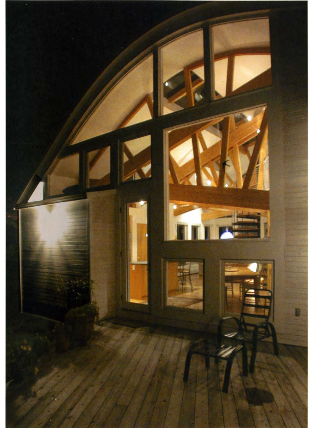
Interior lighting fills the exposed, trussed three-quarter-barrel vaulted space with the activity of architecture.
