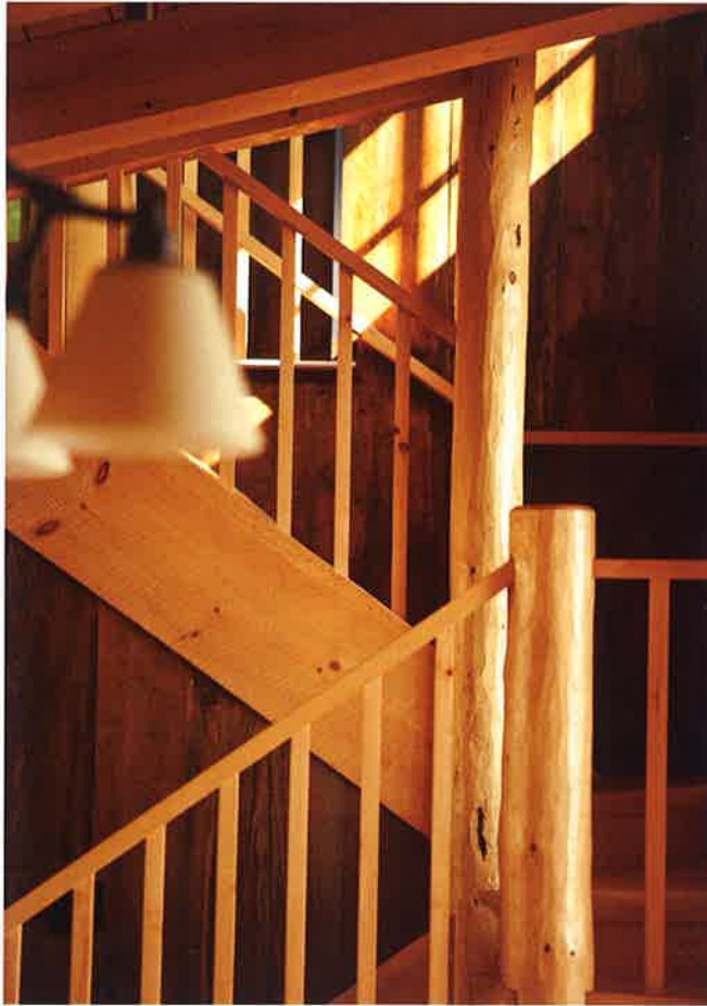
Peeled pine newels (left) echo the house's main support posts and are typical of the unpainted, natural woodwork throughout the building.
