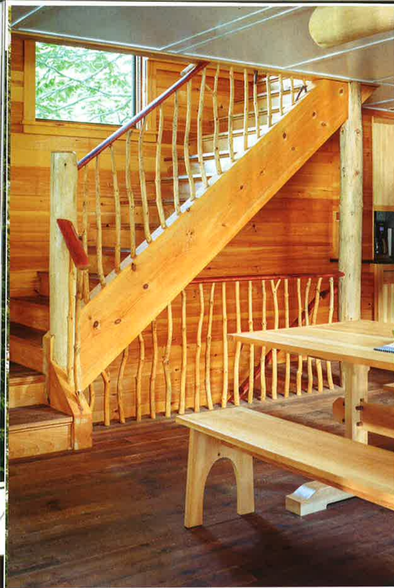
(Above, from left to right) The staircase in the Guesthouse consists of pine logs and branches handpicked from builder Nate Holyoke's Bucksport property.
